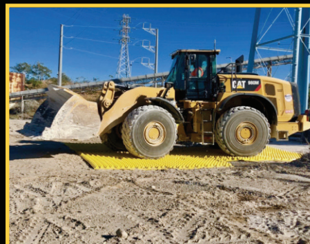
● Industrial Gypsum Plant
